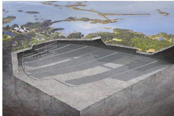
Spent Fuel Repository at Forsmark
