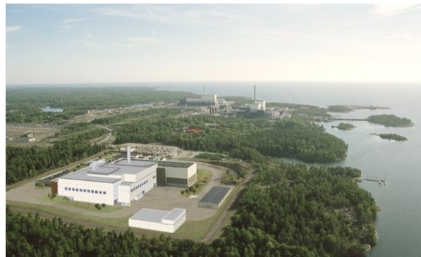
Encapsulation plant in Oskarshamn
