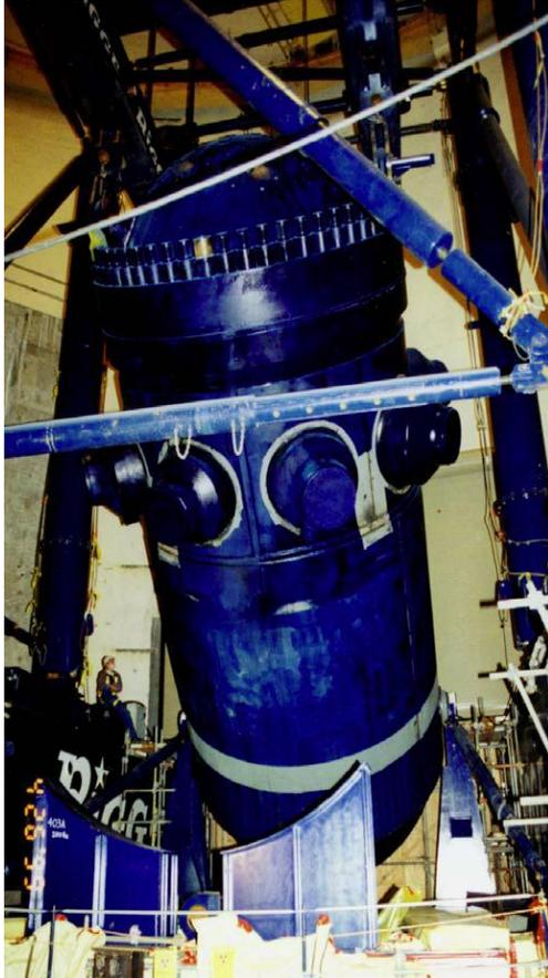
Figure 2-3 Preparation of the RPV Outside the Containment Prior to Shipping
