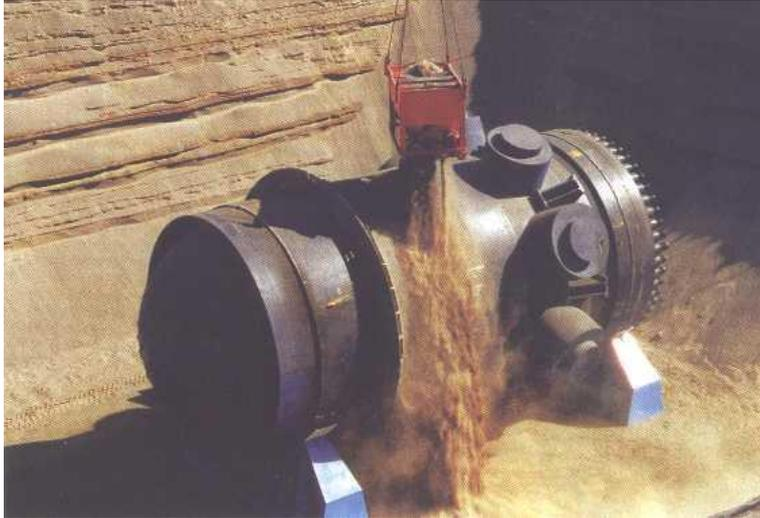
The approach to this part of the project was based on the assumption that, if the reactor internals could be inserted into the RPV and the RPV back filled with concrete, the radioactivity contained in active metal would be calculated over the entire volume of the RPV. The RPV and internals together contained 74.37 E15 Bq of activated metal.
