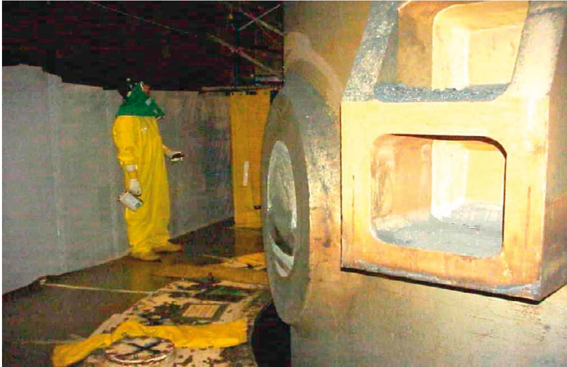
Figure 7-3. San Onofre Unit 1 Reactor Vessel Nozzles after cutting with a diamond wire saw.
