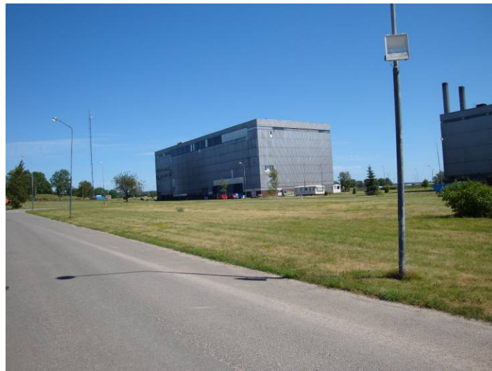
Figure 2-19 External View on Old Sorting Facility
