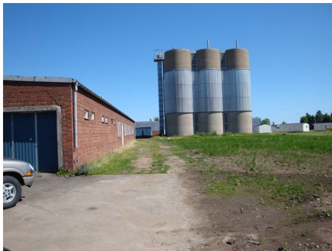
Figure 2-24 Control Building with Lime Silos in the Background
