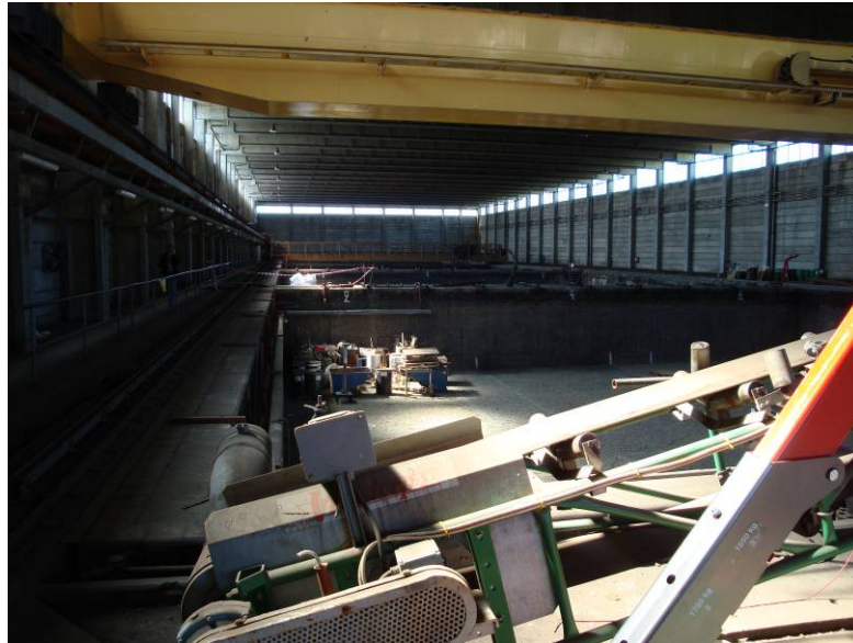
Figure 2-2 Interior Overview of Large Leaching Hall Pools
