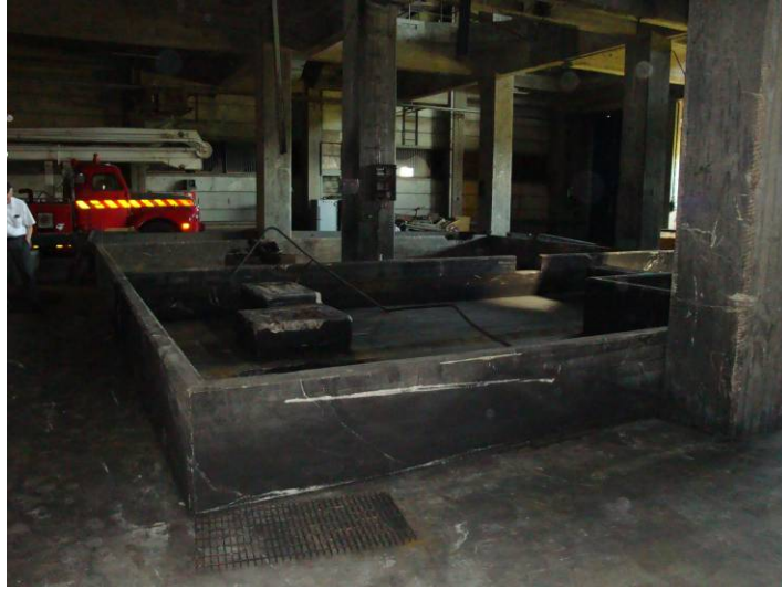
Figure 2-20 Magnetite Slurry Pools in Old Sorting Facility
