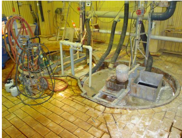
Figure 2-9 Tanks Used in Second Stage of Flocculation Process
