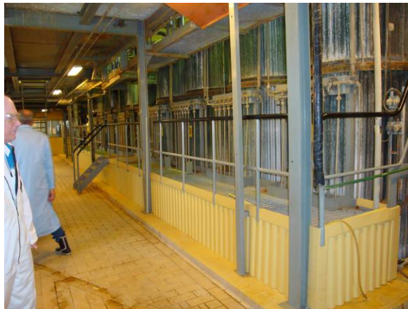
Figure 2-14 Mid section of Percolation Leaching Vessels
