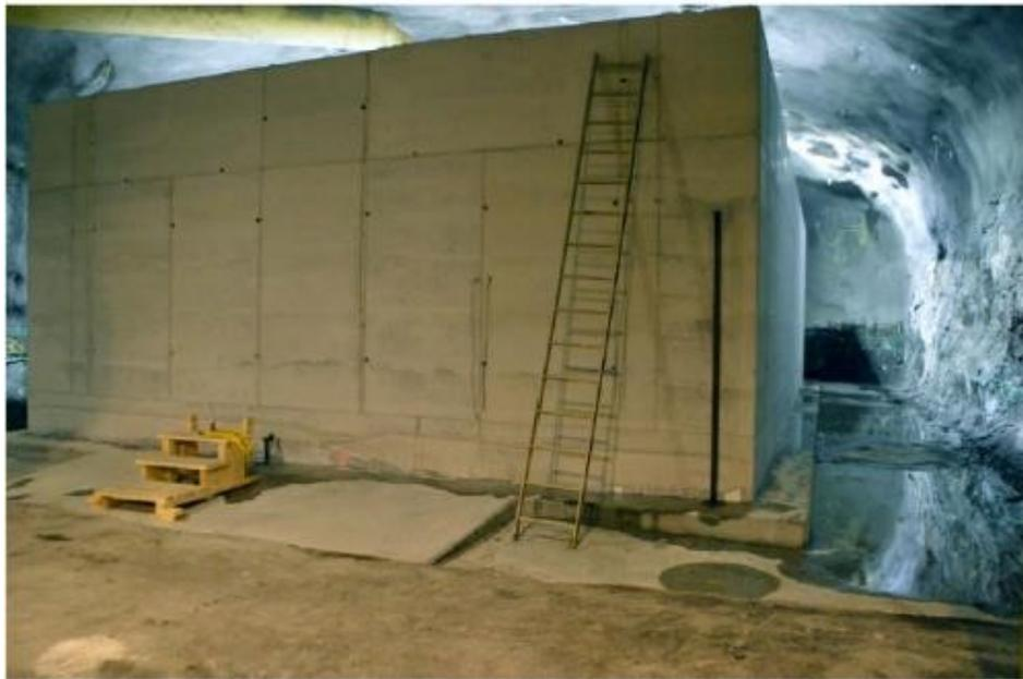
**Figure 16:** The caisson after formwork removal (SKB TR-20-09)
