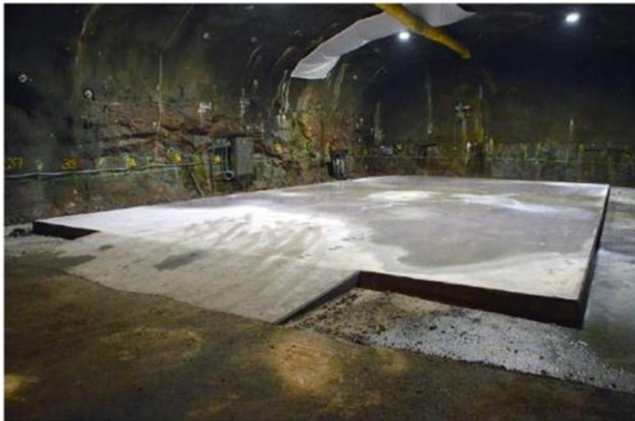
**Figure 10:** Final surface finish once the test area was complete (SKB TR-20-09).
