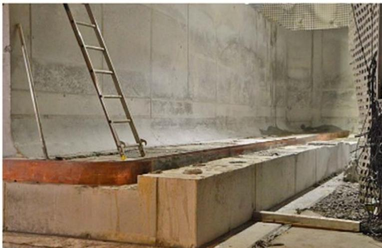
**Figure 6:** Section 1 after removal of formwork (SKB TR-18-12).
