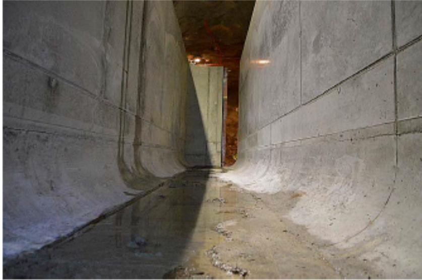
**Figure 8:** Interior of the trial structure with Component 2 on left and Component 1 on right. Water in base from groundwater leakage from tunnel roof (SKB TR-18-12).
