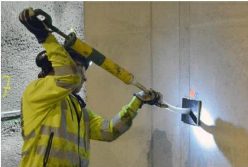
**Figure 18:** Grouting hole with hand-held injection pump (SKB TR-20-09).
