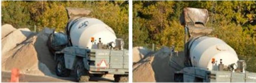
Figure 5-10. Feeding aggregates (0-4 mm) into the truck mixer:
