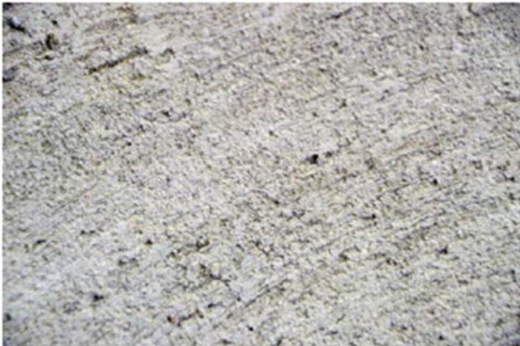
**Figure 15:** Coarse surface finish of the base slab, indicating tearing of the drying surface during trowelling (SKB TR-20-09).
