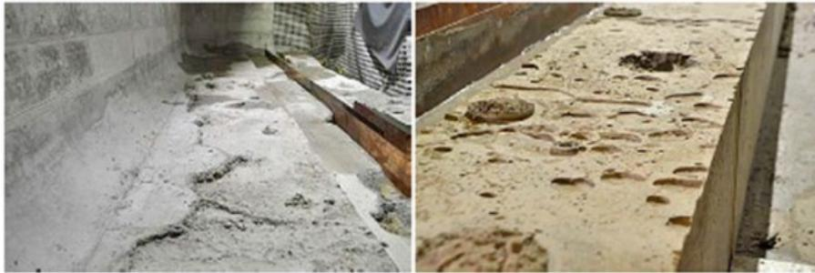
**Figure 5:** Images showing imperfections on surface of the base slab (SKB TR-18-12).
