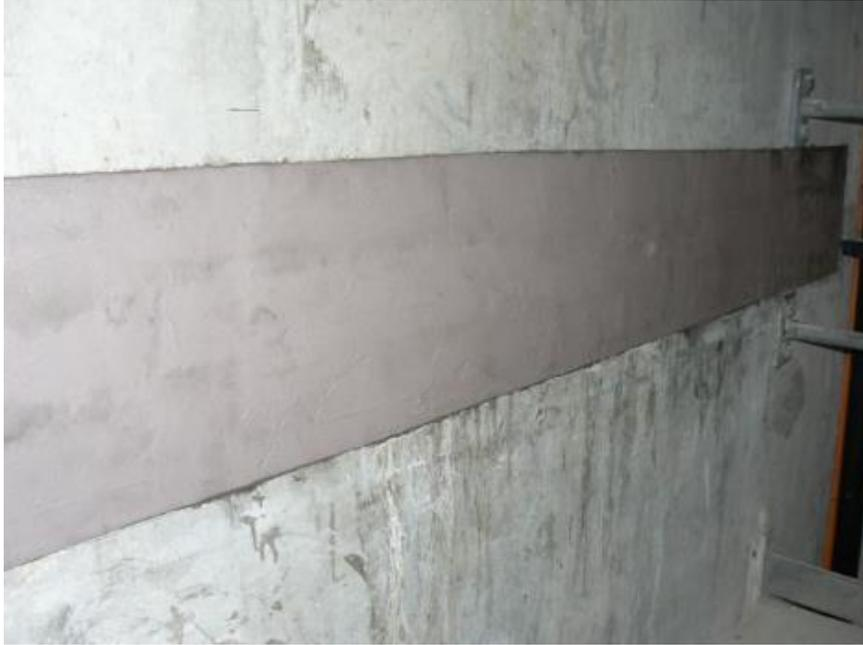
**Figure 35:** Application of high-quality cementitious coating on horizontal construction joint.
