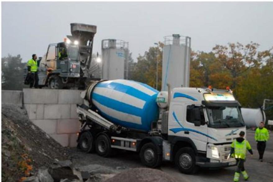
Figure 13: Truck mixer positioned for pouring concrete into the transport truck (SKB TR-20-09).
