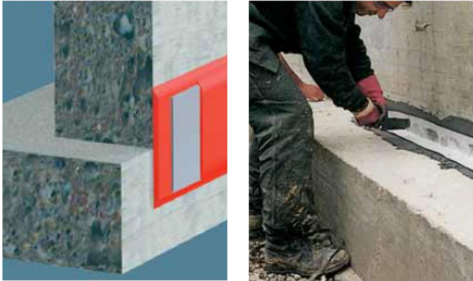
**Figure 34:** Example design and installation of high-quality joint waterproofing.
