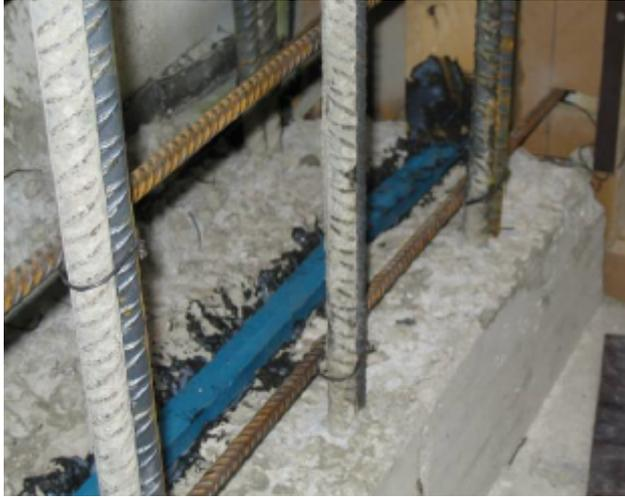
**Figure 31:** Hydrophilic waterstop in position on top of an integral kicker.
