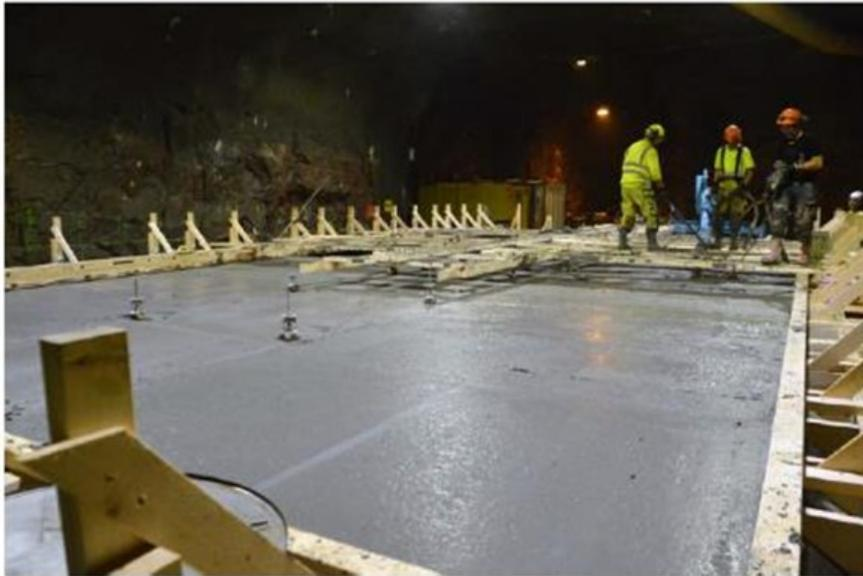
**Figure 14:** Base slab formwork ready to receive concrete (SKB TR-20-09).
