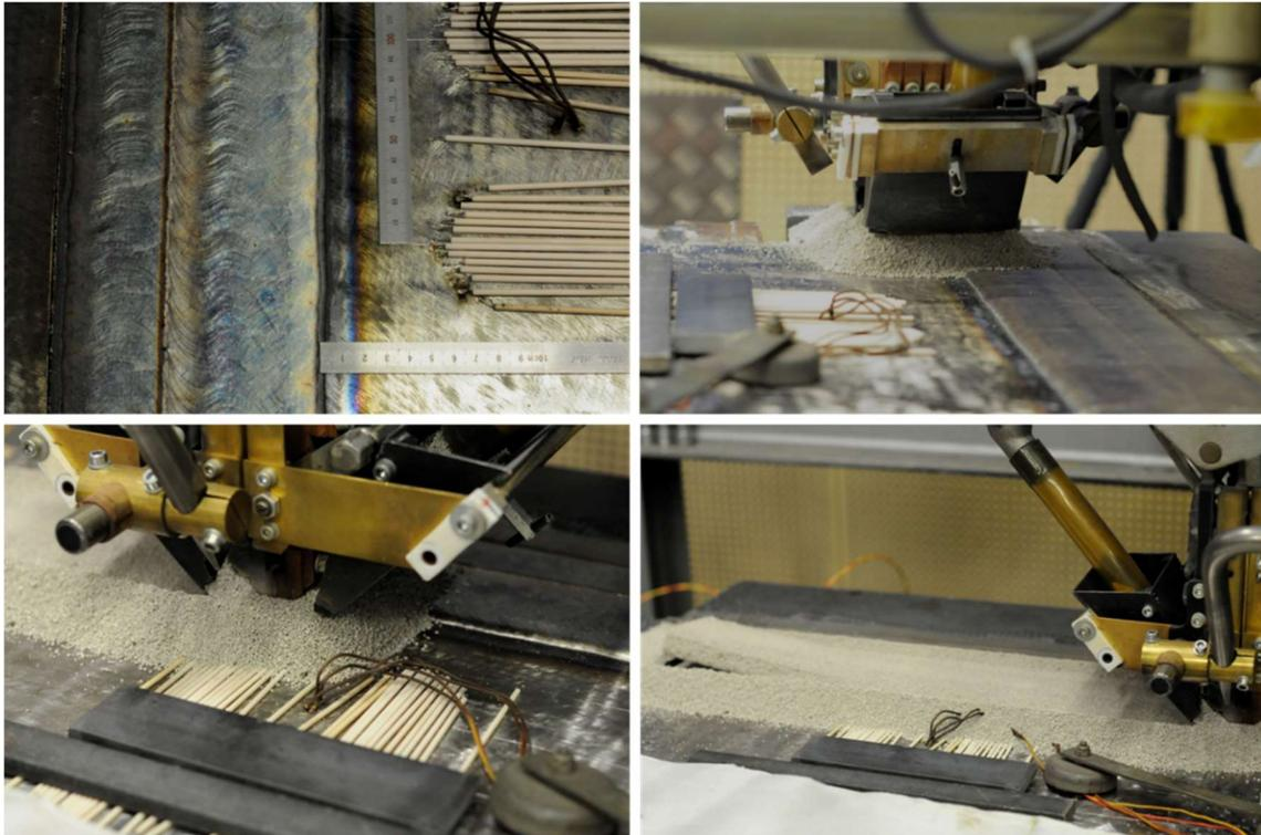
Figure 5 Submerged arc welding of cladding strip #3 on the mock-up. Thermocouples are also seen in the pictures.
