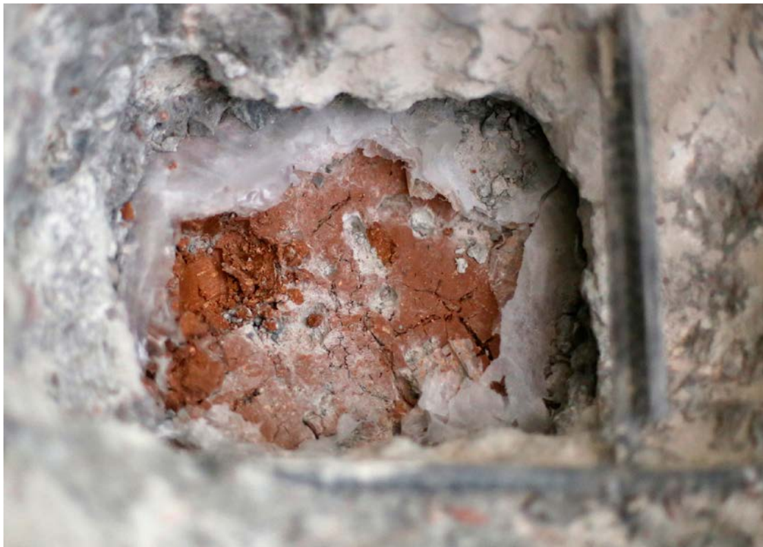
Figure 2-14. The silo bentonite as it looks in 2014. Picture is taken through a hole in the temporary lid.
