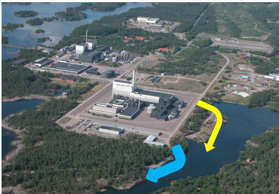
Figure 1-5. Oskarshamn NPP with the cooling water outlet for unit Oskarshamn 1 and 2 in yellow and for Oskarshamn 3 in blue. The outlet into Hamnefjärden is on the north side of the Simpevarp peninsula.
