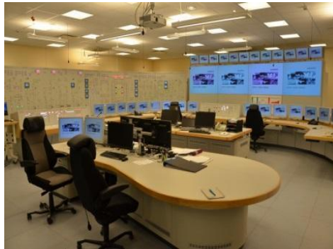
Figure 13. OKG O2 control room simulator.
